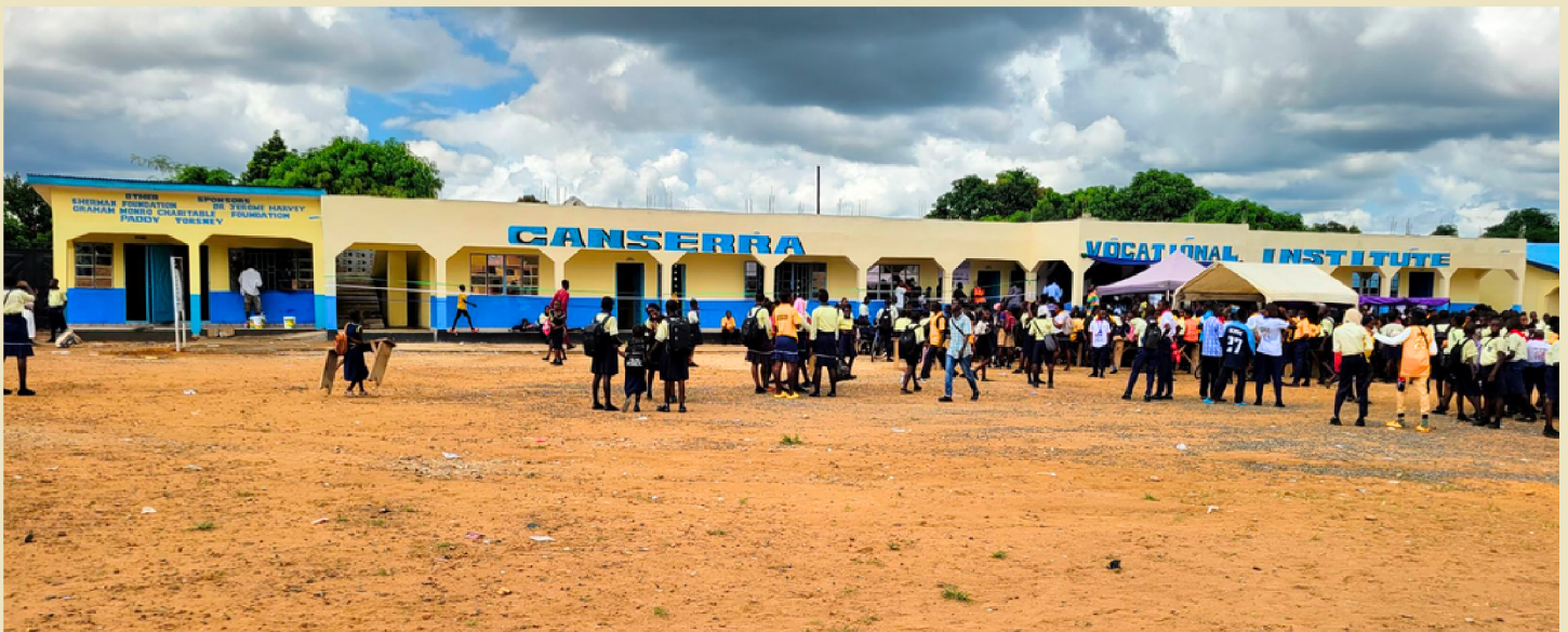
The newly constructed CanSerra Vocational Institute in Waterloo, Liberian Camp, Kissi Town, Sierra Leone.
